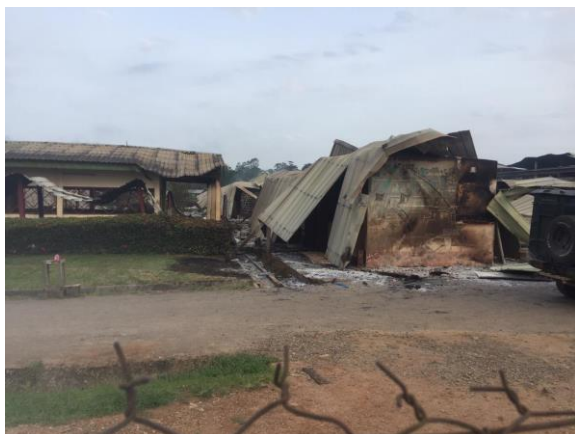
Mamfe district hospital after it was destroyed Credit: partner
